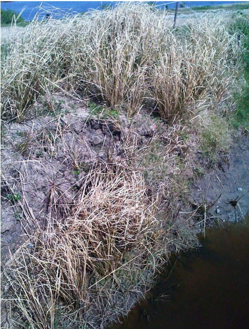
the bottom row of Vetiver, slid down because the bank sheared off. The bank is very steep here, going down to a depth of about 2 meters
